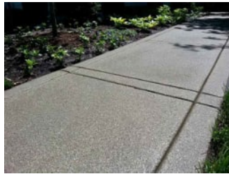
CONCRETE SIDEWALK WITH MEDIUM SAND FINISH
